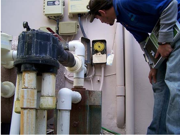
Indexing valve and mechanical timer... a MDC classic!
