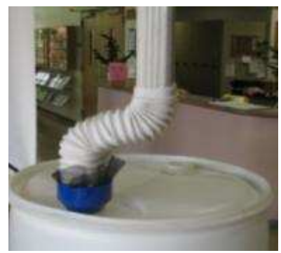
Using Bung Holes with PVC Pipe Increaser
